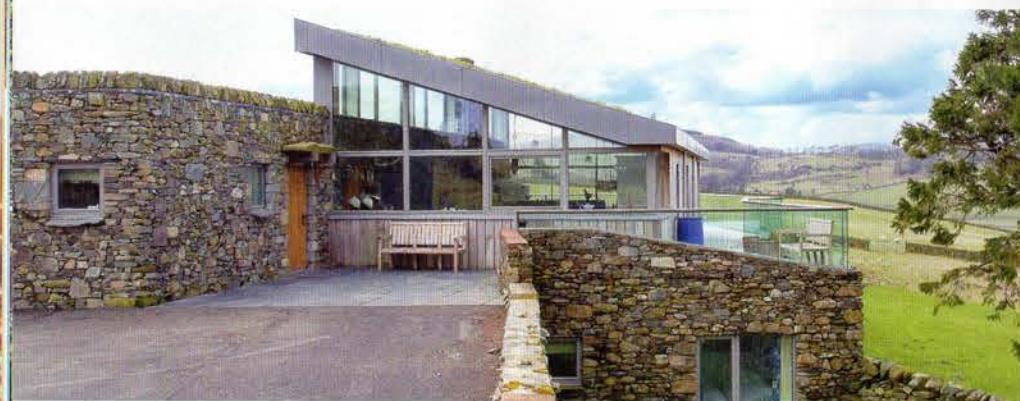
The random stone cladding, which was sourced on site, echoes the dry walling that reaches out on either flank
