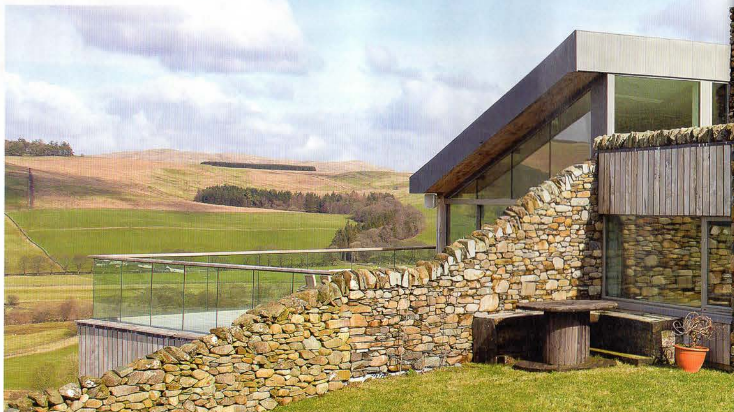
The random stone cladding, which was sourced on site, echoes the dry walling that reaches out on either flank
