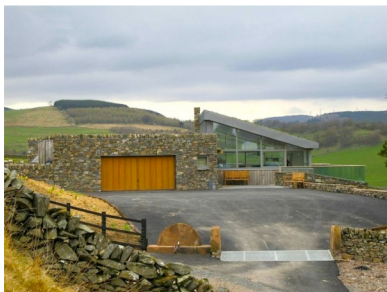
Three Glens in Scotland is built mostly from materials found on the farm. Image via Mark Waghorn Architects.
