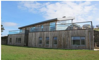
The oak paneling comes from trees on site and the wall insulation comes from the farm's own sheep's wool. Image via Mark Waghorn Architects.
