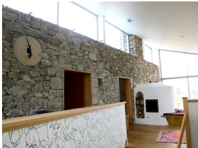
The walls come from locally found stone and the rooms are heated by a wood-fired kachelofen stove. Image via Mark Waghorn Architects.
